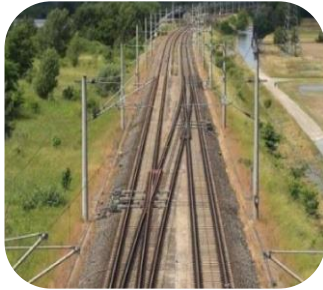
2. Street trees, railroad greens
