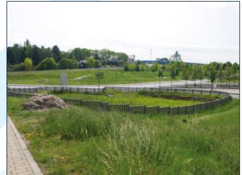
Natural Rainwater retention basin
