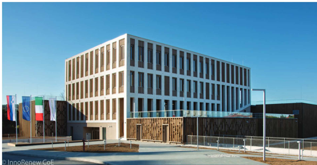
Image 9: The new building of the InnoRenew CoE institute is an example of activities that are compliant with the values of the New European Bauhaus; furthermore, it also boasts the title of the largest timber building in Slovenia. Incorporating sustainable construction principles, it has been shaped to create a better user experience (Source: innorenew.eu ).
