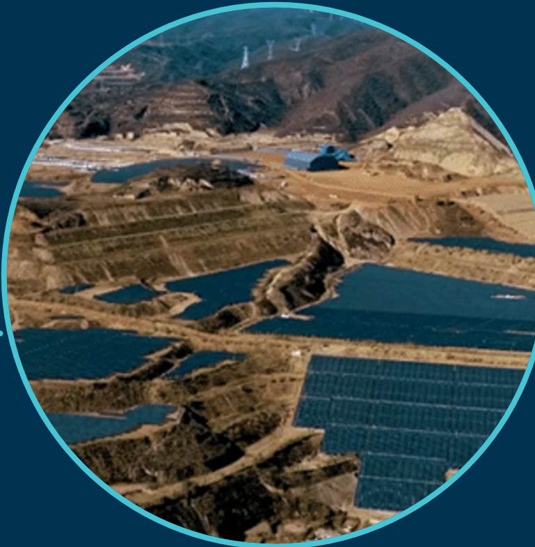
PV panels on mining benches
