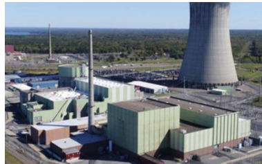
Nine Mile Point, US, In Operation hydrogen generation
