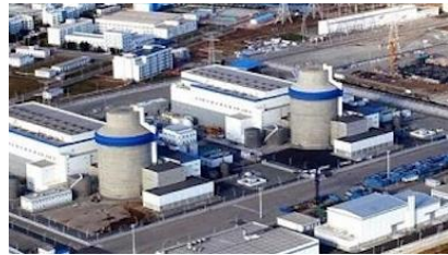
Haiyang- China AP1000 In Operation (District Heating)
