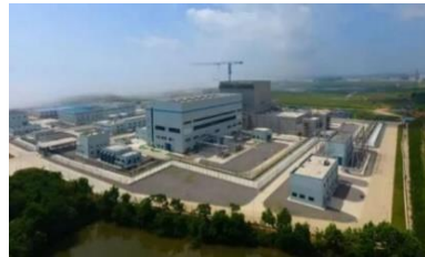
HTR-PM, China, High Temperature Reactor in operation
