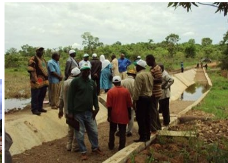
A small dam in Fètèkou in Benin rehabilitated
