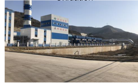
VAM destruction plant with 25 MW steam turbine to generate electricity Working Mine, Yangquan, Shanxi, China
