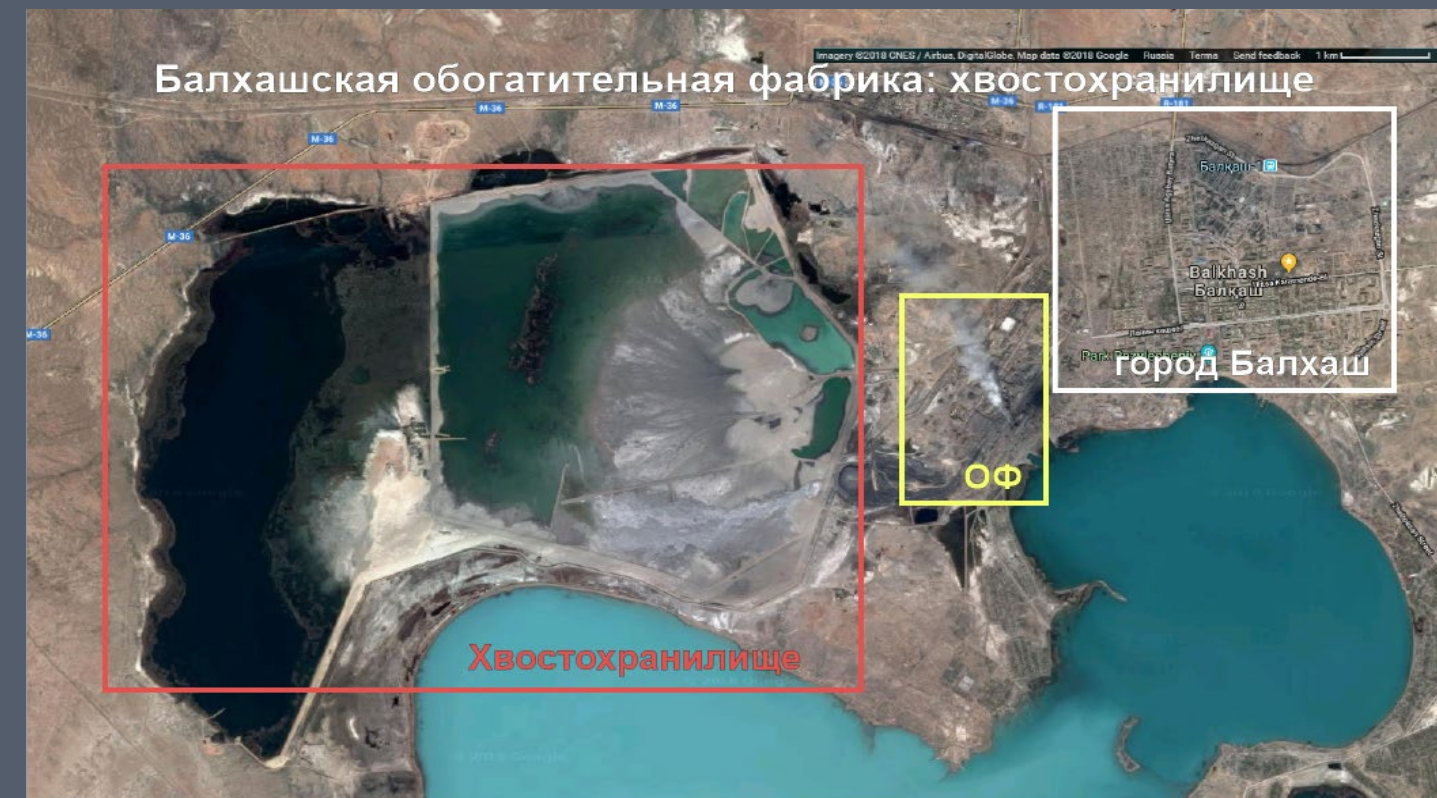
TMF of the Balkhash ore dressing plant
