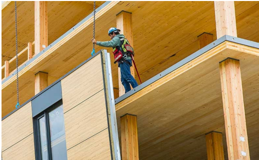
Wood in construction works
