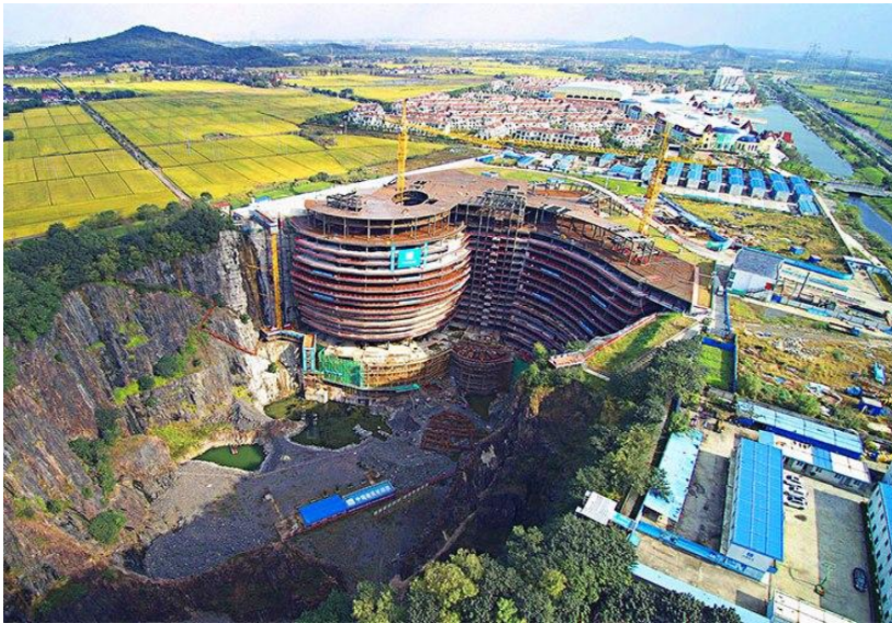
Deep Pit Hotel during construction, Shanghai (Martin Jochman, credits: www.china-underground.com )
