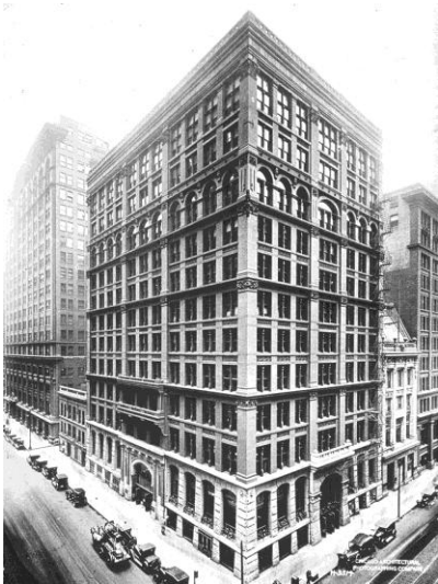
Chicago, Home Insurance Building (William Le Baron Jenney, 1885, torn down in 1931, credits: Wikipedia, Chicago Architectural Photographing Company)
