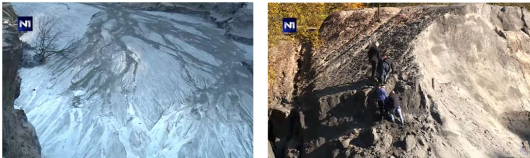
Stolice tailings dam collapse after heavy rain, Serbia, 2014
