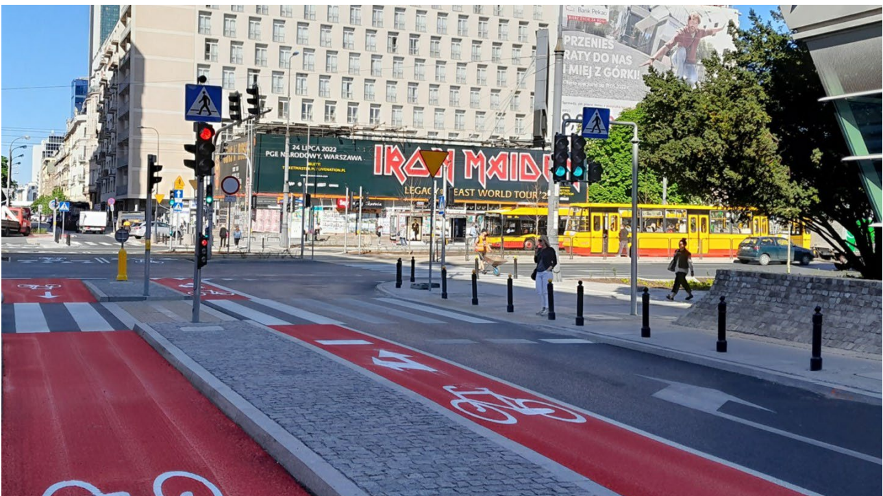
Figure 1. The traffic light signal on the left side is meant only for cyclists, and in line with the current wording of the convention includes a silhouette of a cycle. But with the traffic light lit it is almost indistinguishable from the traffic light for cars (rightmost one). Source Aleksander Kopiński
