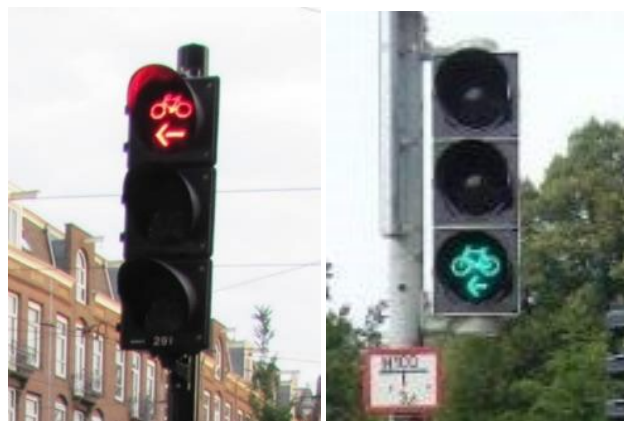
Figure 5. Traffic light signals for cyclists turning left in Netherlands (left) and Germany (right).
