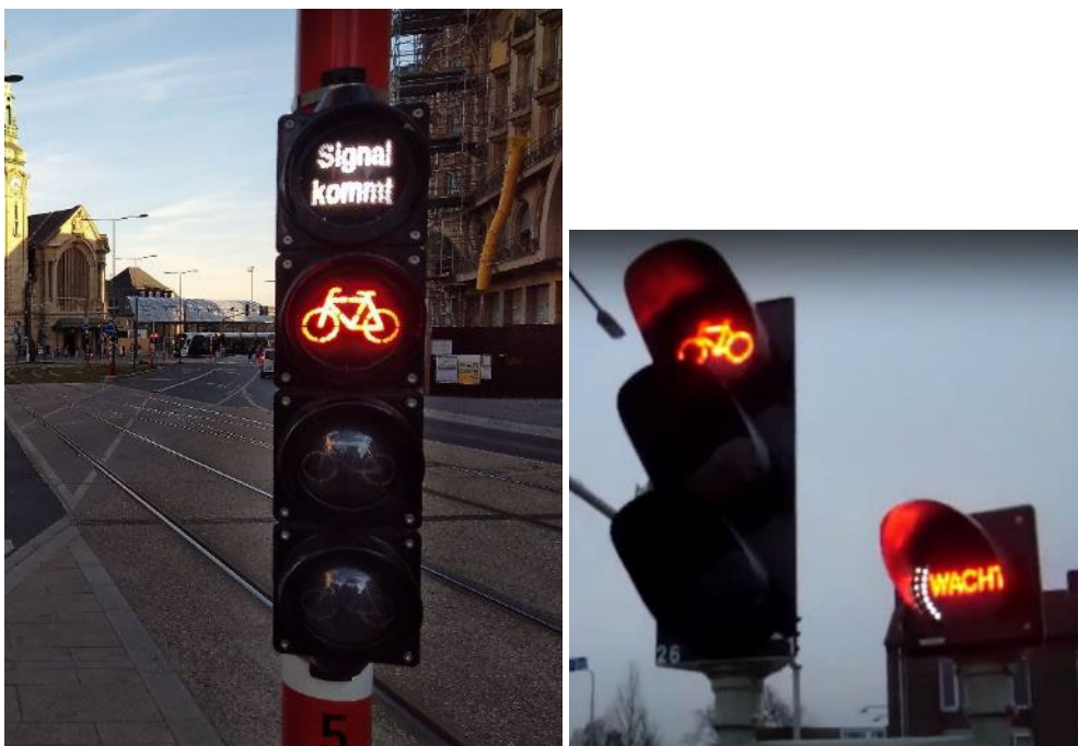
Figure 7. Detection confirmation in Luxembourg (left); detection confirmation combined with an estimate of waiting time in the Netherlands (right).
