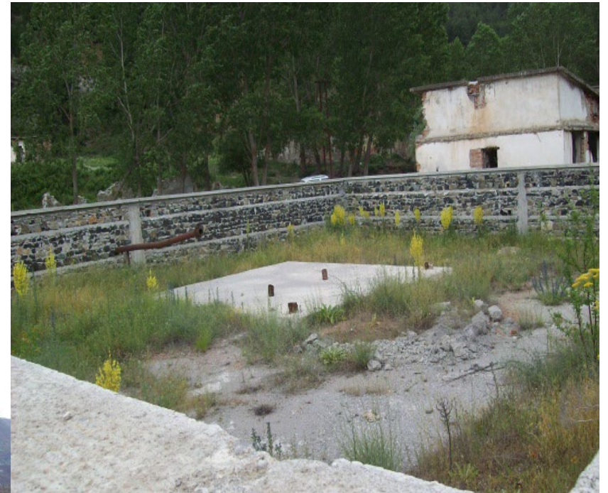
Closed and Rehabilitated well
