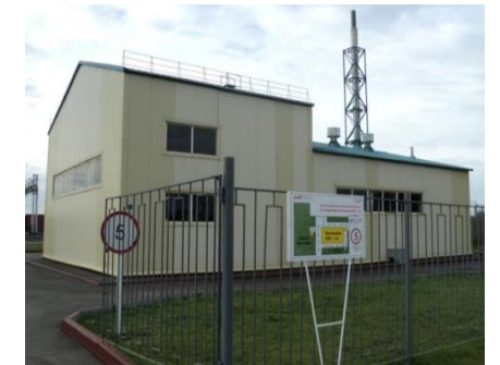
Catalytic cogeneration plant-based boiler facility
