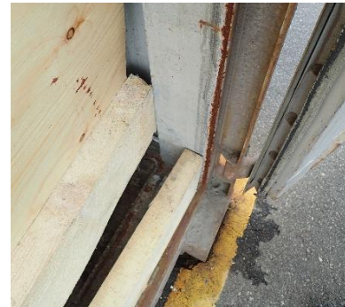
Figure 7.73 Beams too short
