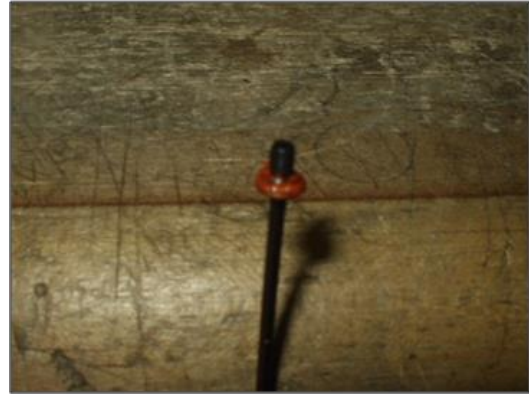
Figure 34 Add sealant to the cover screw
