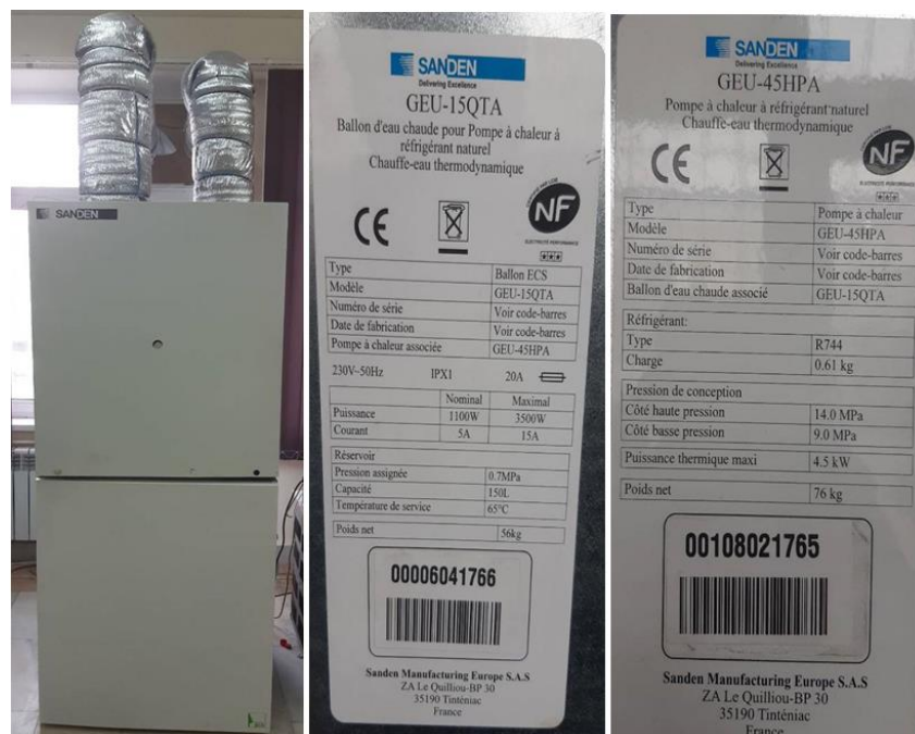
Figure 13. Air-to-water heat pump operating on an environmentally-friendly CO 2 refrigerant (R744)
