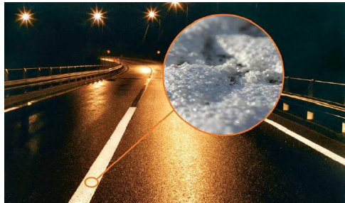
Type II markings (wet-night visibility)
