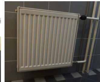
Panel radiators in sanitary facilities
