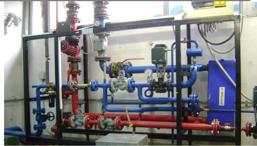
Indirect type of district heating substation in the basement of the nominal heat power 250 kW (manufacture date 2000.)
