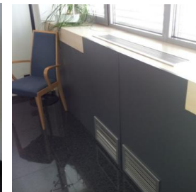
Vertical exposed and concealed two-pipe fan coil units
