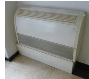
Vertical exposed and concealed two-pipe fan coil units
