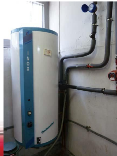
Indirect type of district heating substation in the basement of the nominal heat power 250 kW (manufacture date 2000.)
