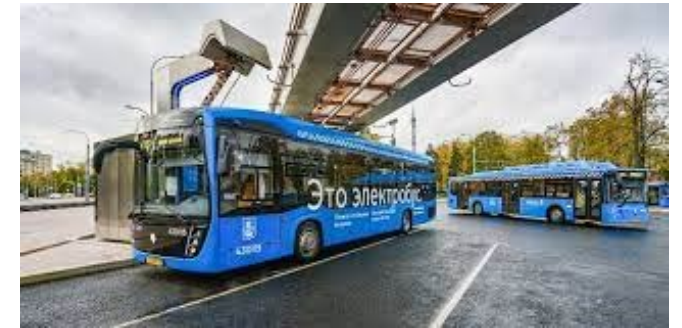
Opportunity charging at terminals
