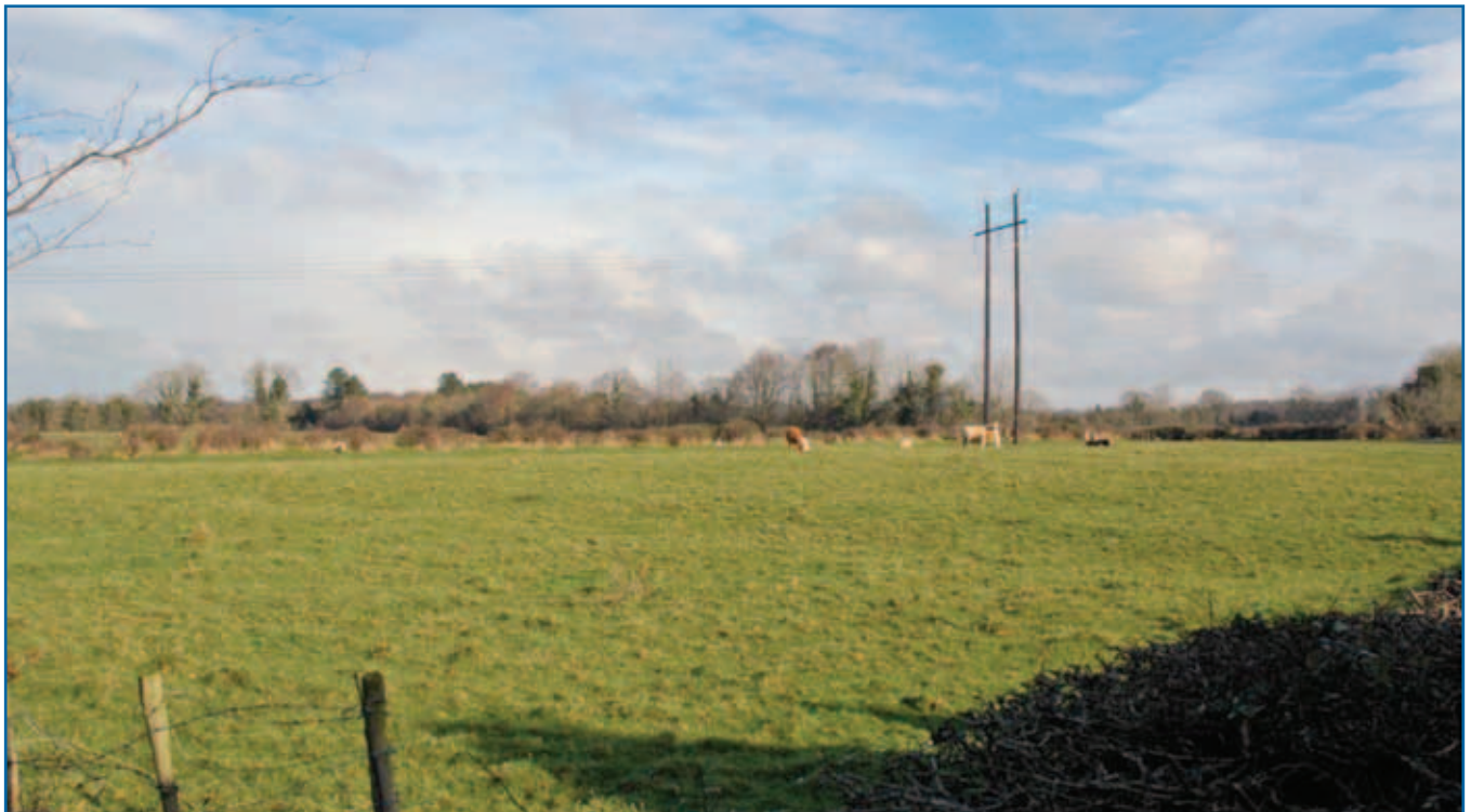
Figure 4: Photograph of a Single Circuit 110 kV wood poleset structure
