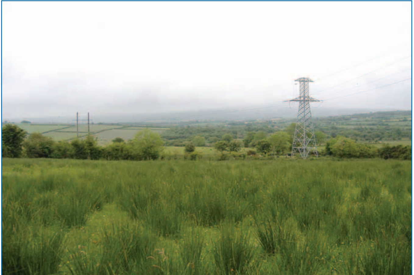
Figure 5: Photograph of a typical Single Circuit 110 kV angle tower structure
