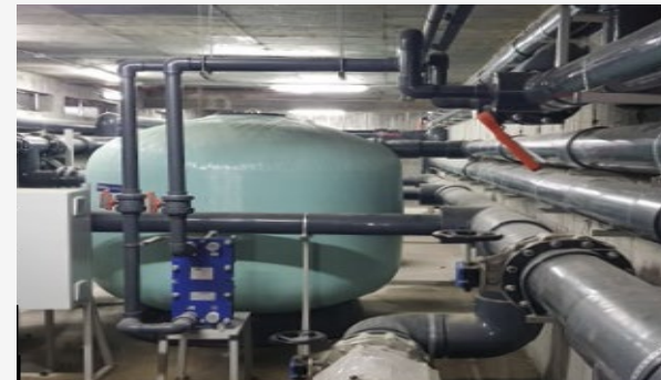
Completed subsurface installations of the aqua park, 2019 (courtesy of N. Toholj)
