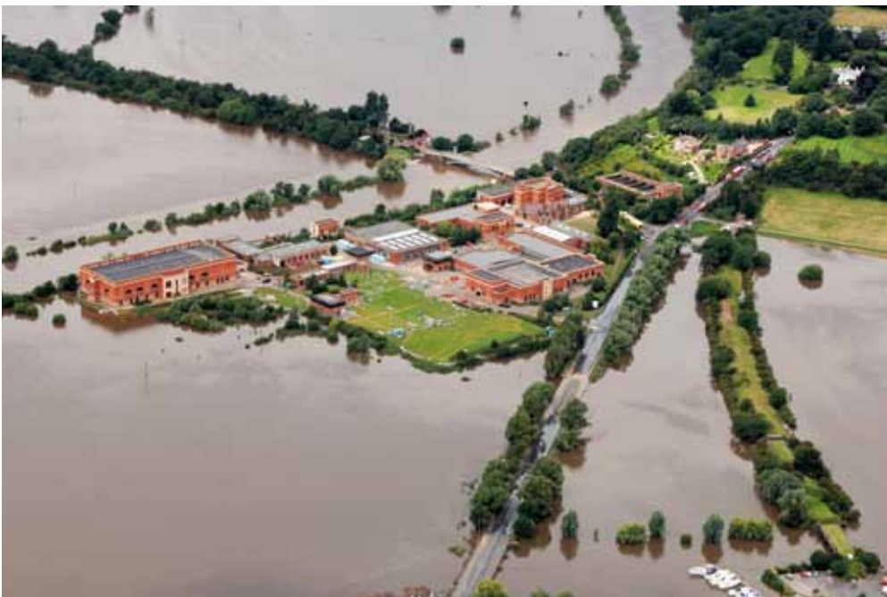
Flooded drinking-water treatment plant, Mythe, Gloucestershire (United Kingdom), 2007 © British Geological Survey
