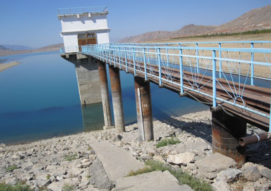
Tortgul Reservoir: Pre-rehabilitation of equipment (2009) © GIZ archive
