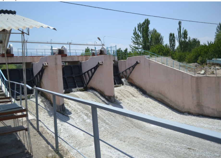
Zumratsho Headwork: Post-rehabilitation (2014) © Umed Komilov
