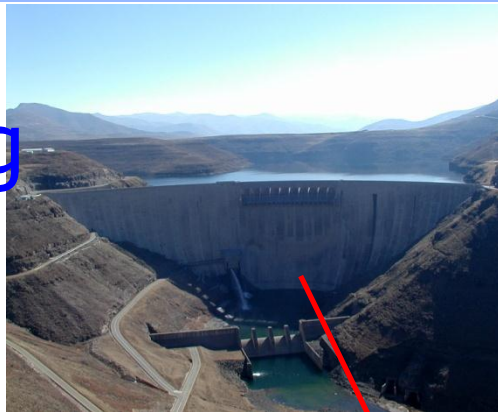
Khatse dam - Orange river
