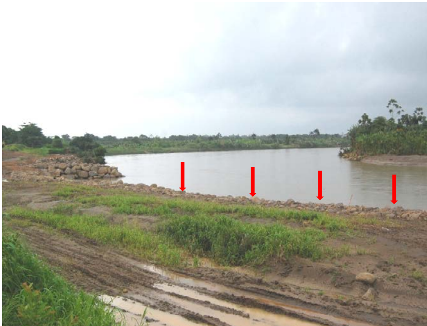
Retaining wall against flooding. To the right, banana plantations ( Panama )
