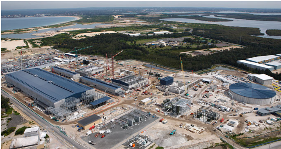
Desalination plant in Sydney, Australia
