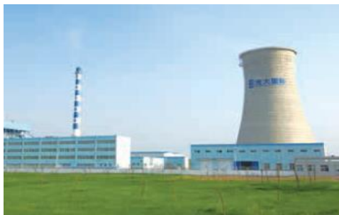
CEI: Dangshan Biomass Power Project (BOO)
