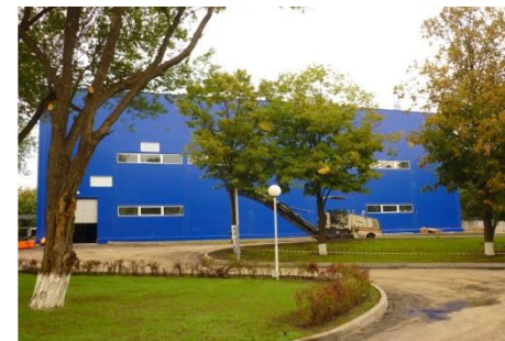
Construction of 3 ultraviolet units at WTP
