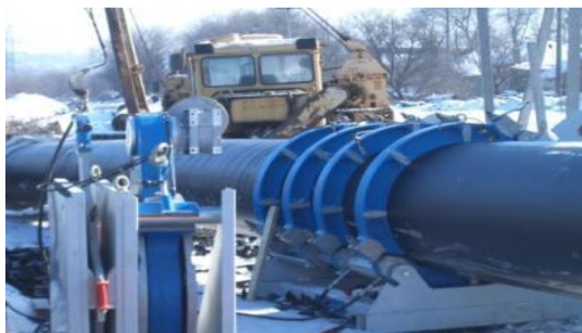
Building of new water mains (41,7 km)
