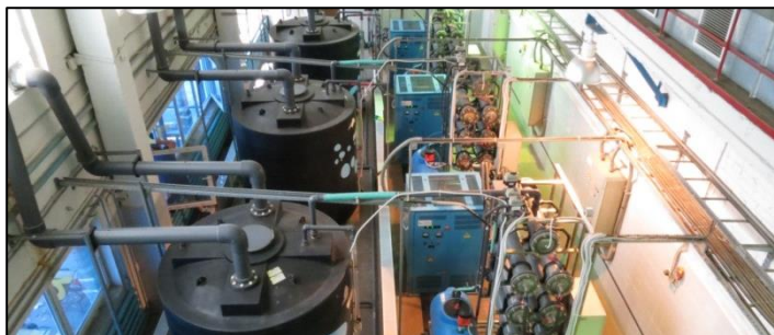
Reconstruction of the biggest WTP, replacement of free Cl by NaClO
