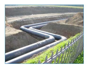
Construction and operation of a network of a district heat distribution from waste burning plant for 8000 houses.
