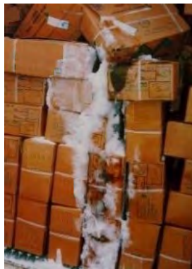
Figure 1.12 Ice from leak in door gasket
