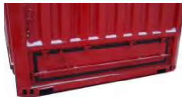
Figure 3.43 Letterbox type hatch in container front wall
