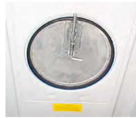
Figure 9.11 Roof hatch internal lock
