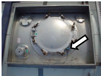
Figure 9.14 Manway hatch seal
