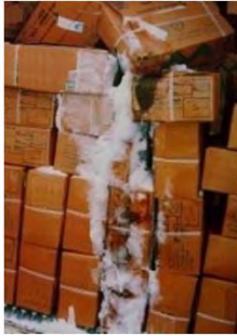
Figure 4-12 : Ice from leak in door gasket
