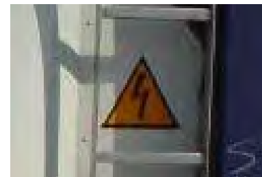
Figure X-5 : Overhead warning sign
