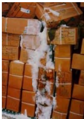
Figure 4-12 : Ice from leak in door gasket
