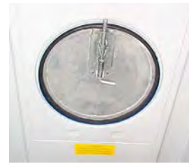
Figure XI-11 : Roof hatch internal lock
