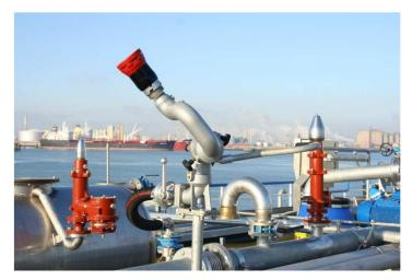
Hydrant point equipped with a jet/spray nozzle – with a hose of sufficient length. Hoses could be replaced altogether by a fixed water line. However, current legislation indicates that a hose has to be present.
