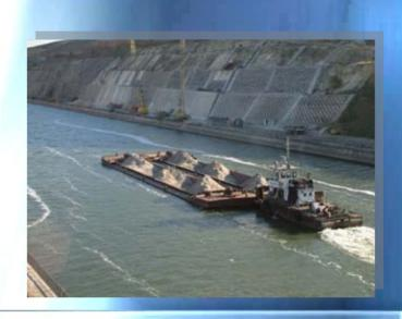
The 64.4 km long and 90 m wide canal has a water depth of 7 m and 17,5 m clearance under the bridges
