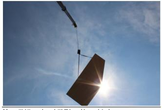
**Note:** CNC-machined CLT board being lifted to its position. **Source:** Schilliger Holz AG, 2012.
