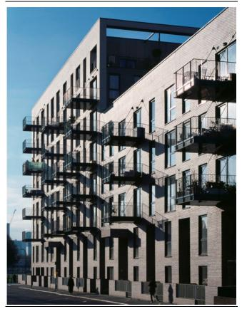
**Note:** 1,198 tonnes of stored CO<sub>2</sub> equivalent: the largest solid timber building in the UK, "Bridport House". **Source:** Ioana Marinescu/EURBAN Limited, 2012.
