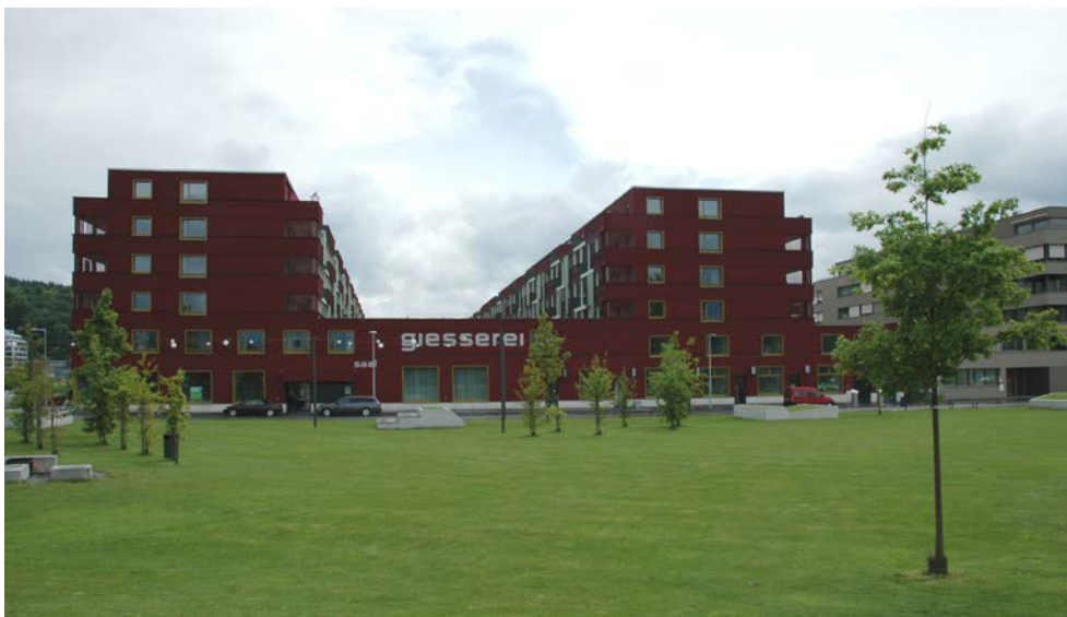
Fig. 3 - “Giesserei” intergenerational residential development (Image source: Michael Meuter, Zürich/LIGNUM)
