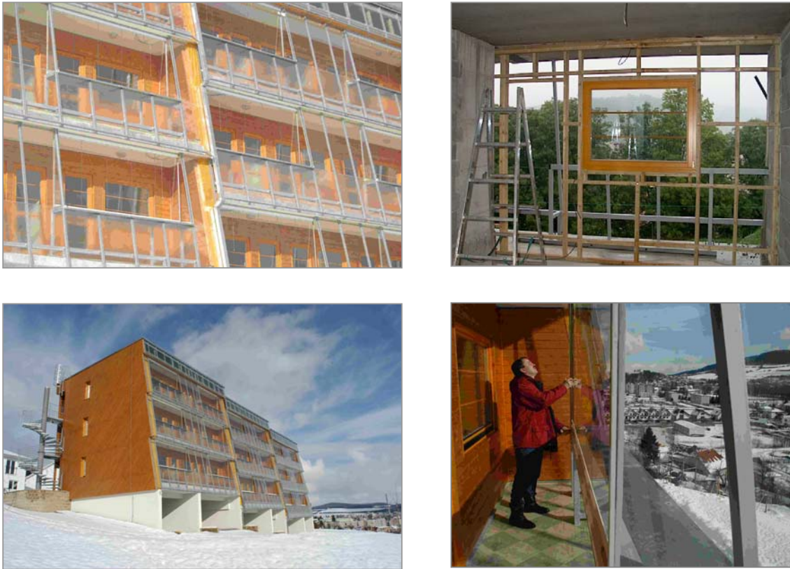
Picture 1 - South-west view and construction details
