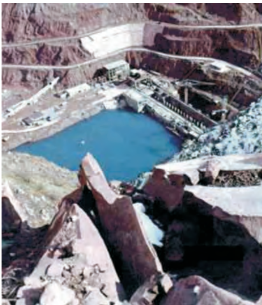
View of the Nurek power dam, Tajikistan.
