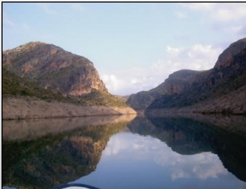
Dam and reservoir inspection
