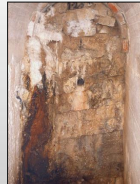
Galleries and foundations
