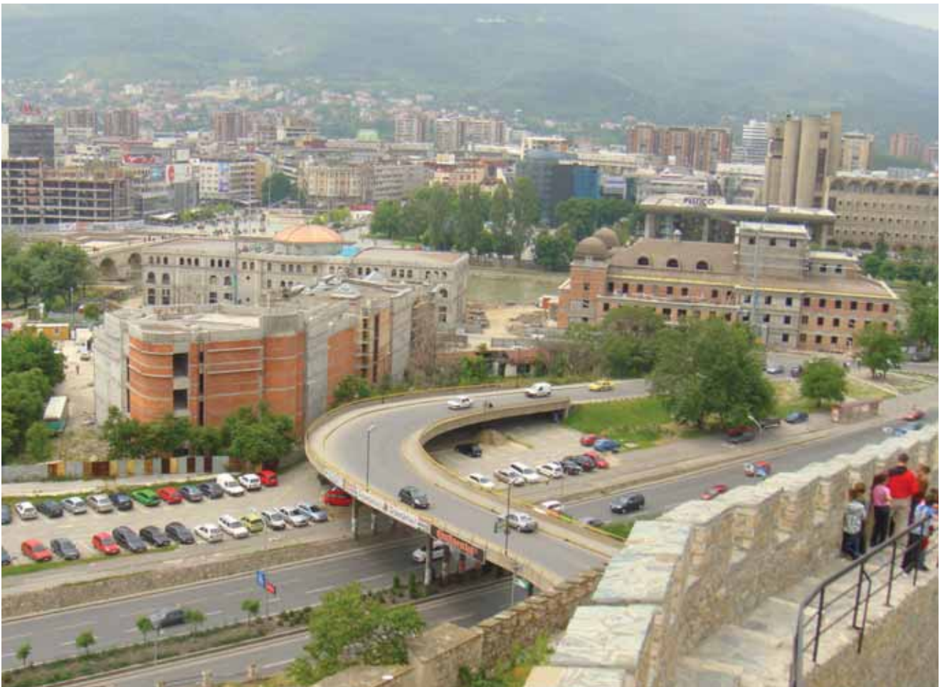
Photo 5.1: Transport infrastructure in Skopje
