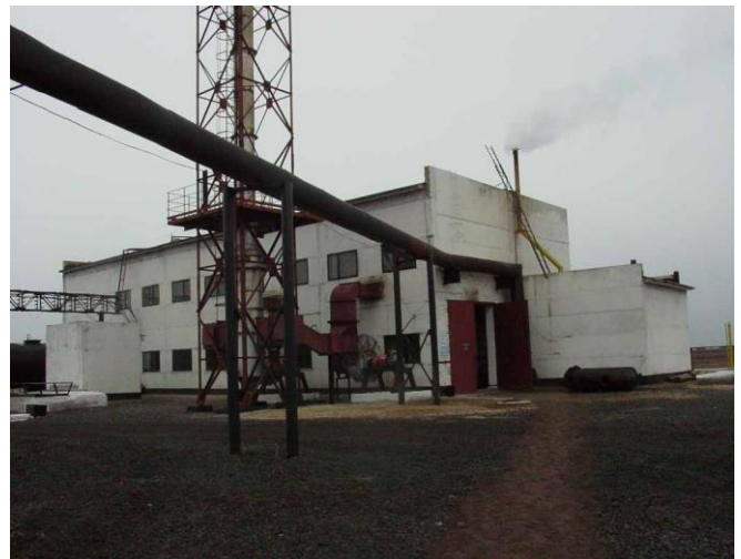
CMM fueled boiler house of AMT - Courtesy of "Industrial Karaganda" and Methane Center PA
